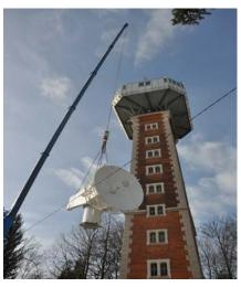
Figure 8: Antenna installed on top of the "Hilmwarte" tower
